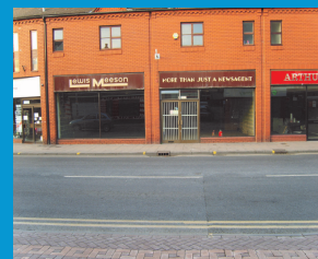
One of the many closed shops and business on Hucknall High Street
