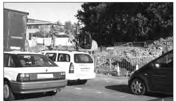
Under way: Work progresses at Segensworth.
