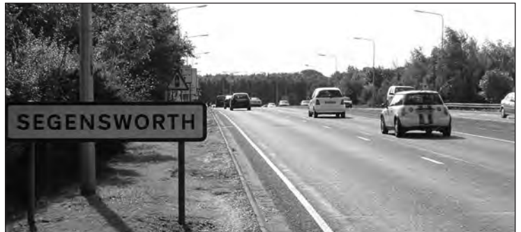
Wider: A fourth lane will be added to the link road from the M27 Junction 9 approach to the roundabout (above).
