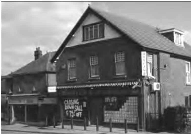
Demolition job: Bastins will make way for even more flats.
