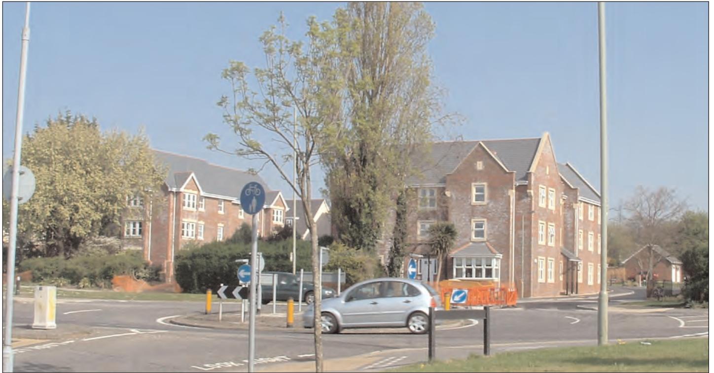
More flats: Several large houses were demolished to make way for this controversial development on Portchester Road at Downend.
