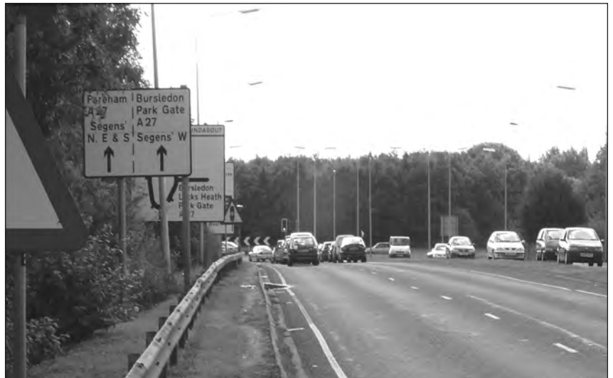
Relief on the way: Work is due to start soon at Segensworth roundabout.
