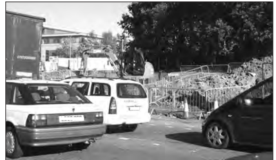
Under way: Work progresses at Segensworth
