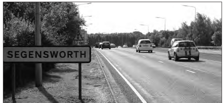
Wider: A fourth lane will be added to the link road from the M27 Junction 9 approach to the roundabout (above).
