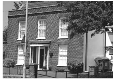
Threatened Listed Town Quay House
