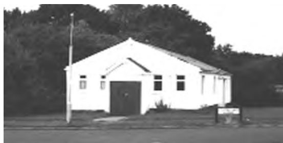
Condemned: Asbestos in the structure was the nail in the coffin for Cams Alders Social Club.
