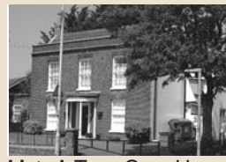
Listed: Town Quay House
