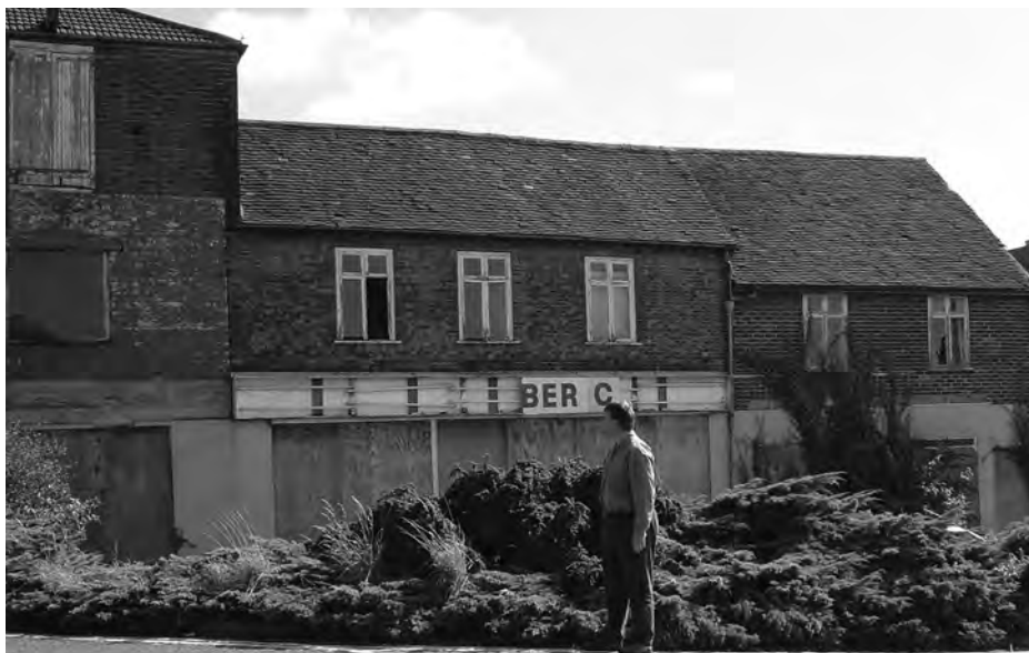
Eyesore: Seán Woodward surveys the foundry site in Quay Street where the council hopes Tesco will build a top class food superstore.
