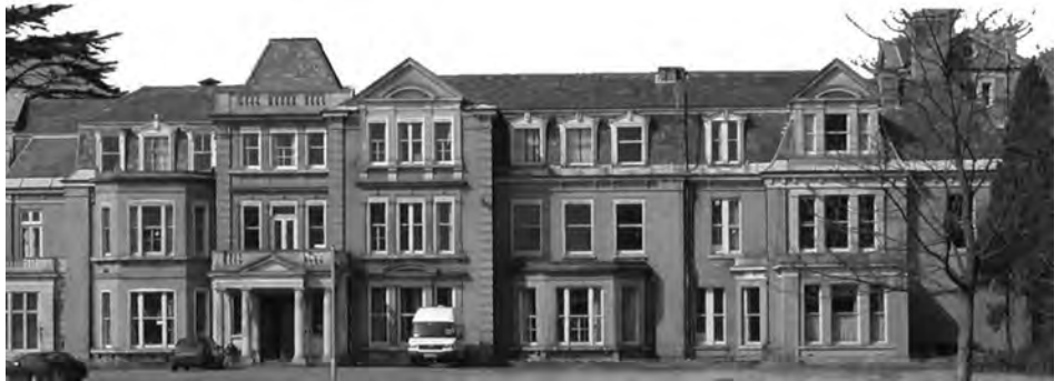
New lease of life: The Council aims to restore and preserve Coldeast mansion (above).
