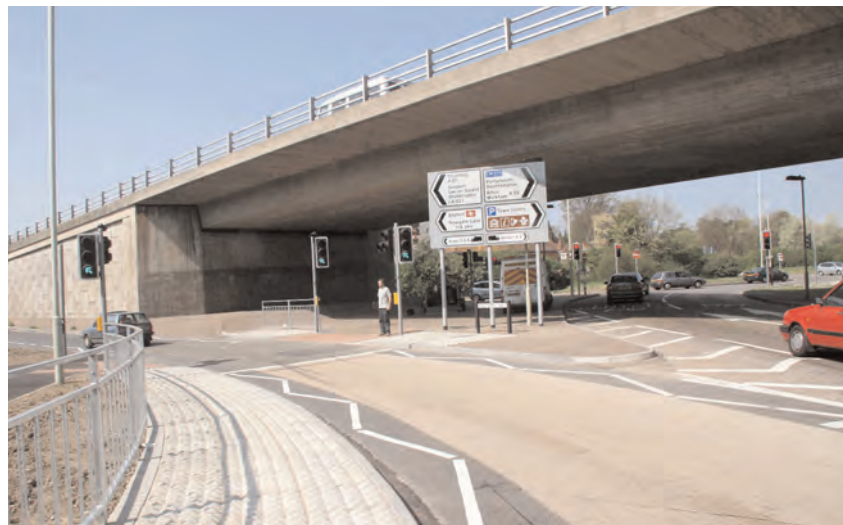
Safety first: The new layout at this section of the Delme roundabout.
