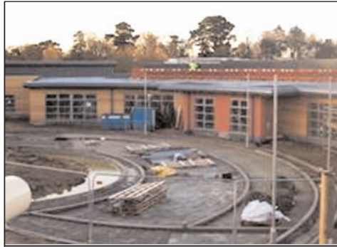
Taking shape: The hospital for which Fareham has waited over three decades.
